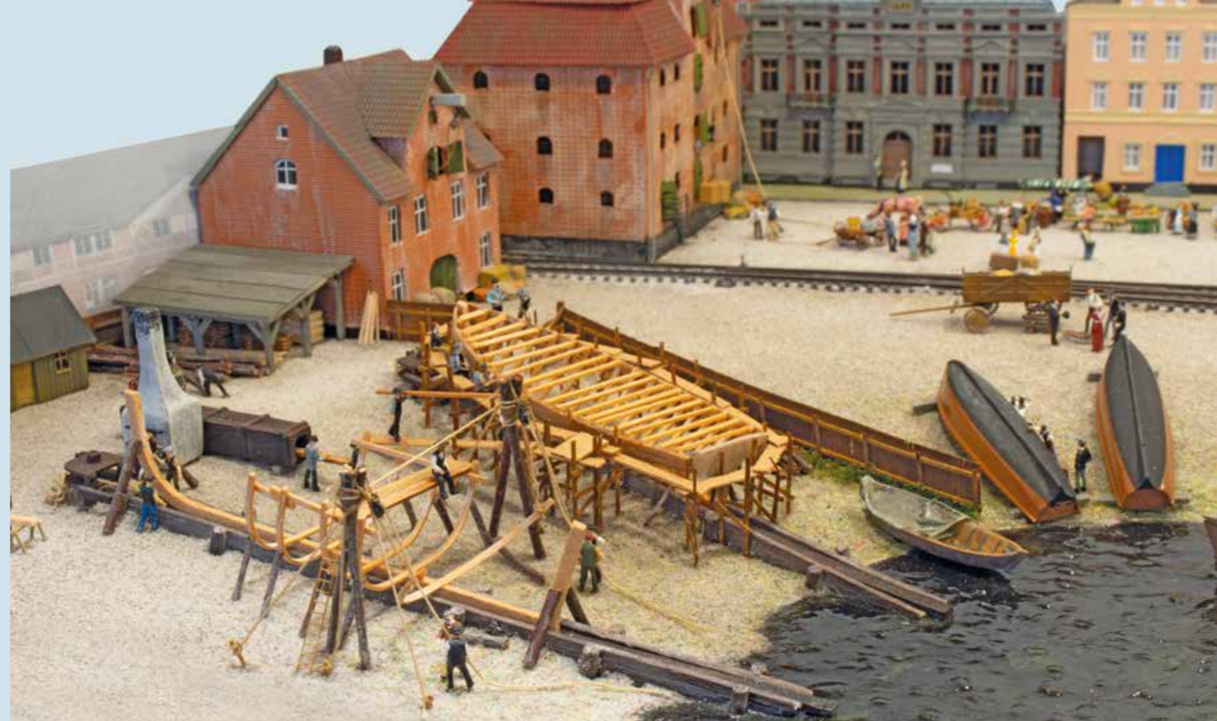
Above Two ships at different stages of construction in the open. Note the steam chamber to make the boards flexible.
